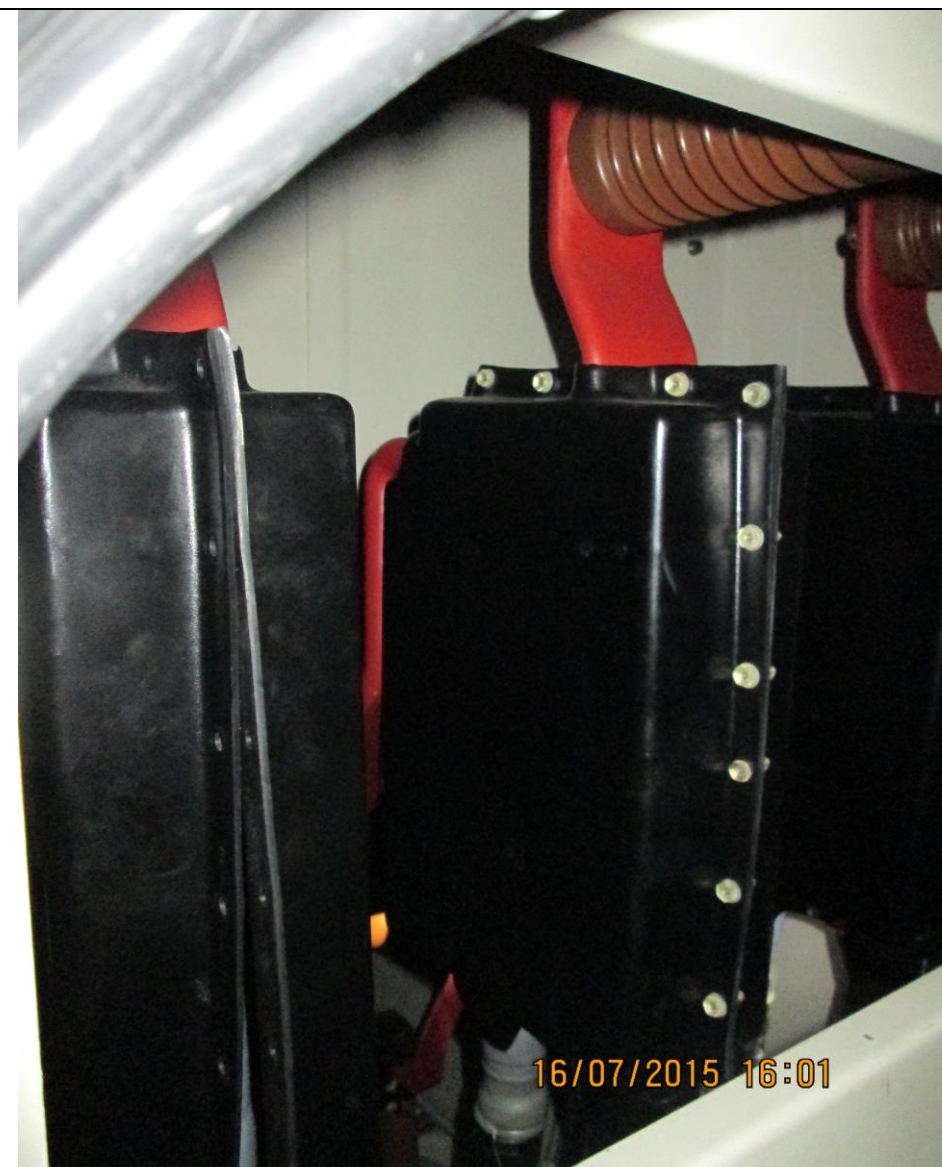
Visible Electrical treeing which originates from the point of touching with cable and the black insulation cover.
