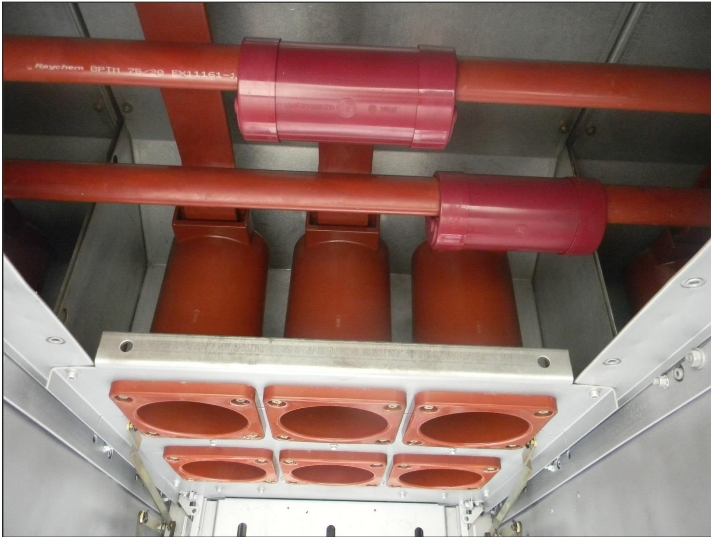
Installed Back Tee Off Bus and New Spouts
